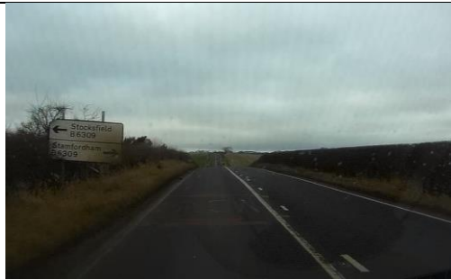
Photo 13 – Worn stack type advanced direction sign which has slipped on posts. Opportunity to improve advanced signage and provide SLOW road markings and red strips.
