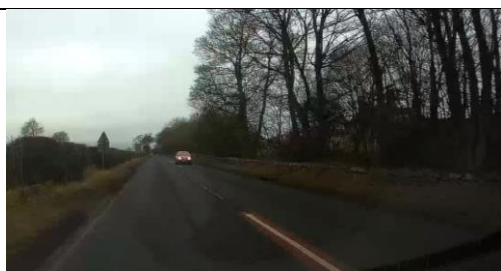
Photo 19 – Example worn set of road markings/studs alongside other markings which have been refreshed more recently.
