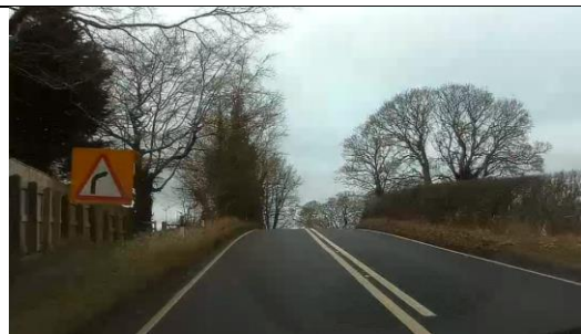
Photo 8 - Example of bend warning sign which could benefit from an appropriate reduced speed supplementary plate
