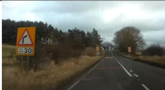
Photo 33 - Example of use of yellow backed warning sign with advisory speed limit. Note however that the advisory speed limit conflicts with the 40mph speed limit terminal signs a short distance ahead.
