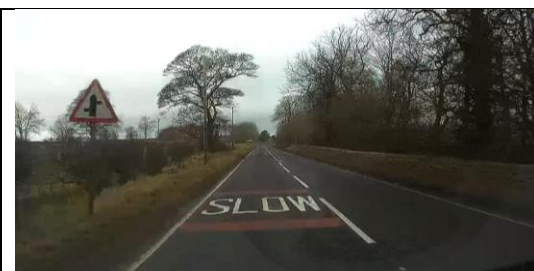
Photo 20 – Example of staggered junction warning sign which could have improved conspicuity and a supplementary distance plate.
