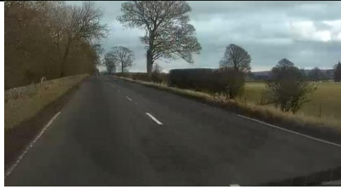
Photo 29 - Example of indistinct road markings beyond another section of road markings which have been refreshed more recently.
