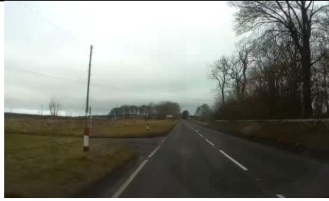
Photo 21 - Example of use of marker posts to highlight presence of minor side road junction.
