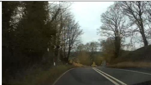
Photo 9 – Chevron sign is hidden within vegetation – suitable clearance required and sign enhanced on yellow backing board.
