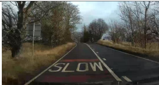
Photo 35 - Warning sign has been twisted to face wrong direction
