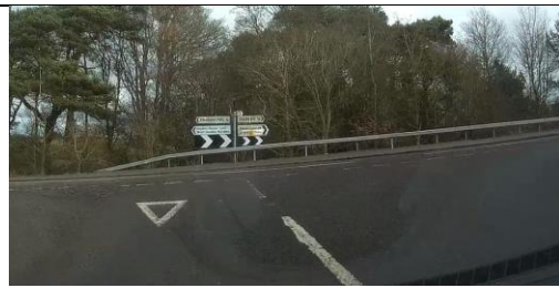
Photo 40 – Chevron “target” signs installed incorrectly. Left chevron should face left or location may appear to be a right bend from a distance.
