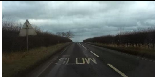
Photo 31 – Warning sign has been twisted to face wrong direction and sign appears worn
