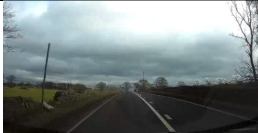
Photo 25 - Missing warning sign (vacant post).
