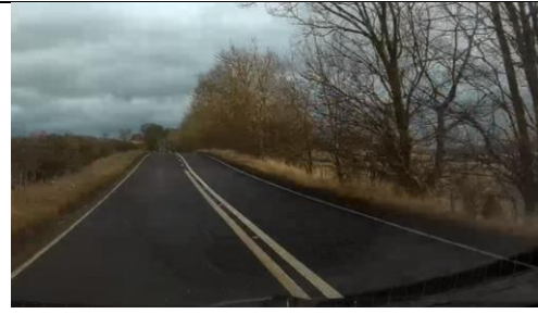
Photo 34 – Check that termination of double white lines and start of broken line is located correctly on an undulating section of road.
