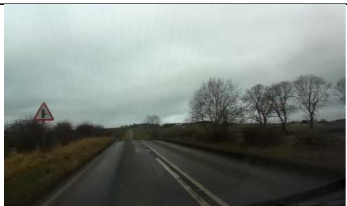
Photo 11 – Ensure termination of double white line system is located correctly, opportunity to enhance junction warning sign and provide SLOW roadmarkings and red surface strips.
