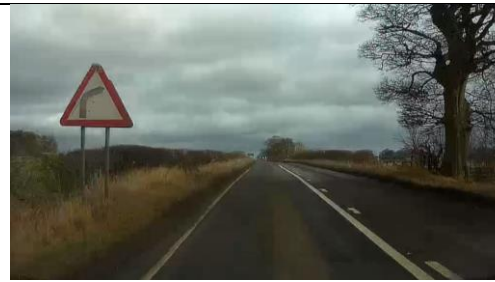
Photo 36 - Example of worn warning sign which could be replaced and enhanced.
