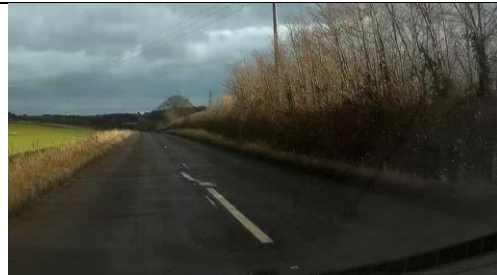
Photo 38 - Example of indistinct road markings beyond another section of road markings which have been refreshed more recently.
