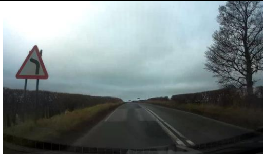
Photo 5 - Example of bend warning sign which may benefit from being located on yellow backing board with a speed reminder.
