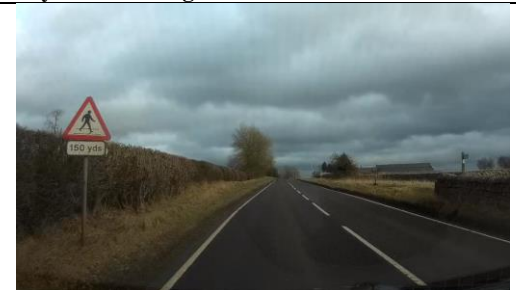
Photo 28 – Incorrect signage in place for a location where pedestrians cross.
