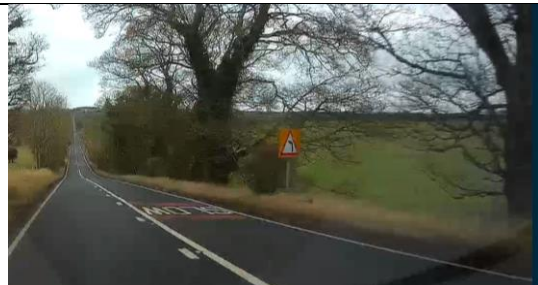
Photo 10 – Warning sign twisted to face in wrong direction and sign may benefit from an appropriate reduced speed supplementary plate
